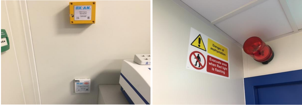
Figure 4 Examples of fixed Oxygen and Carbon dioxide detectors (left) and low oxygen alarm (right) (photo credit: Heriot-Watt University) (ranging from £100-500)
