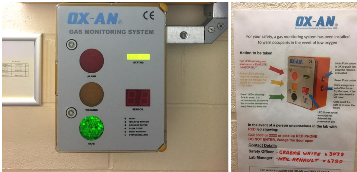
Figure 6 An example of control panel and readouts (left) and instructions next to it (right) (photo credit: Heriot-Watt University) (ranging from £300-5000 excluding electrical engineering cost)
