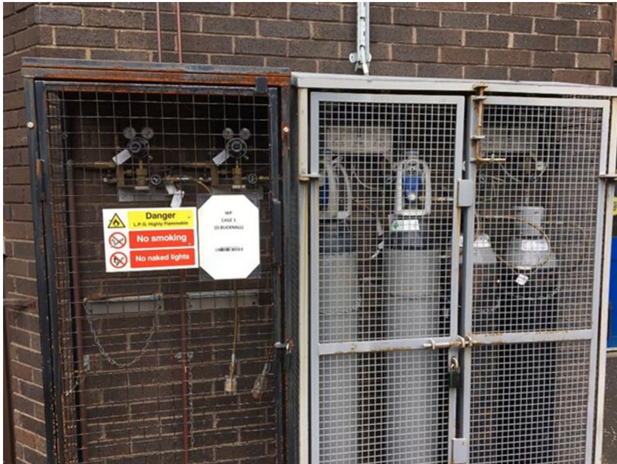
Figure 9 An example of gas cylinder set-up externally to the laboratory (photo credit: Heriot-Watt University)
