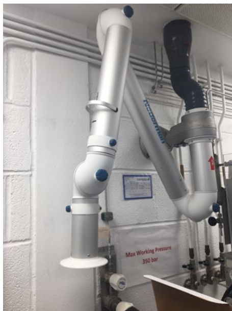
Figure 7 Example of extraction arm for local ventilation (photo credit: Heriot-Watt University)
